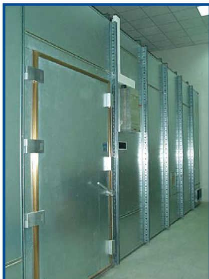
Shielded room example. Exemple de cage de Faraday.
